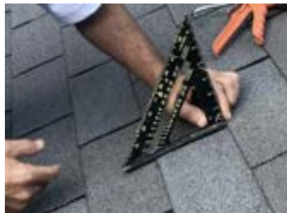
Place square at bottom of the shingle above
